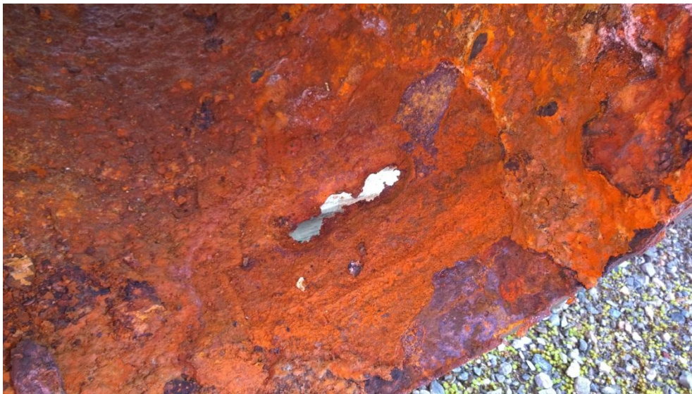
Figure 5: Illustration of Caisson Condition
