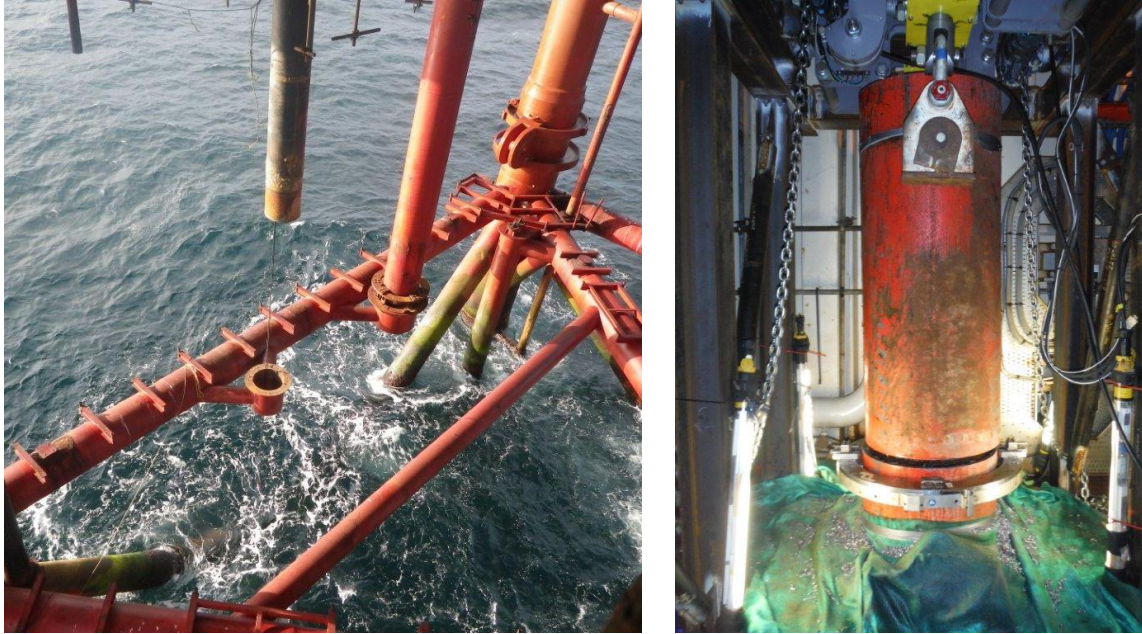
Figure 4: Removal of Caisson
