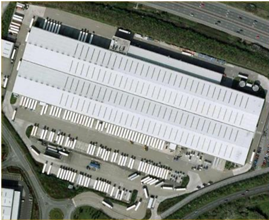
Figure 1: Aerial view of a distribution centre showing lines of closely parked trailers
