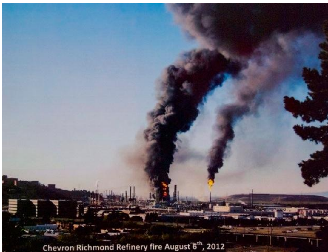
Figure 2 Hydrocarbon plumes due to pipeline rupture (left) and flare (right) at Chevron Richmond refinery (photograph on poster handed out by public interest group during CSB public meeting on April 19, 2013).
