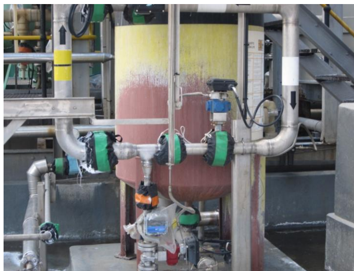
Figure 3: Consistency with standards e.g. taping over of flanges
