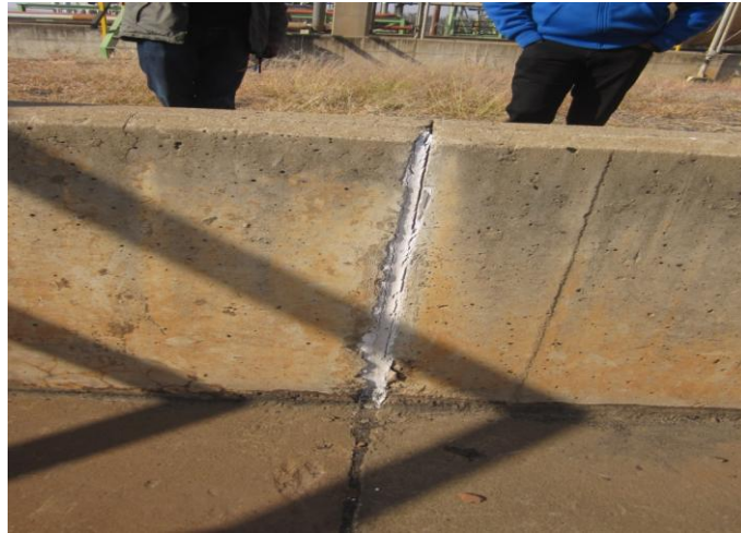
Figure 1: Storage tank bunding condition (sound construction, joint condition, contents)
