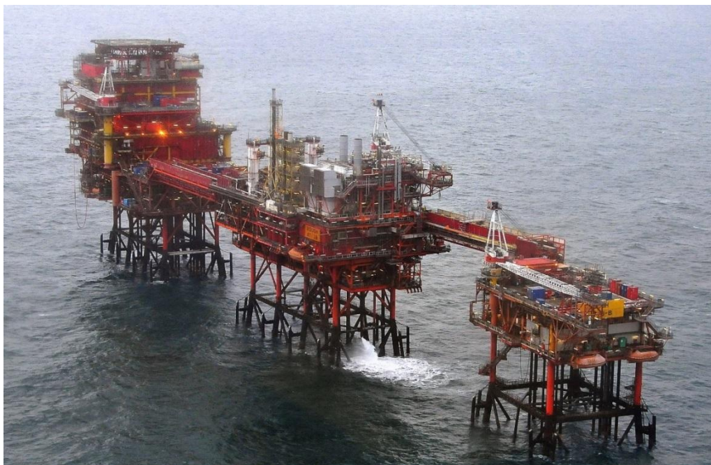
Figure 2. Rough Bravo Installation
