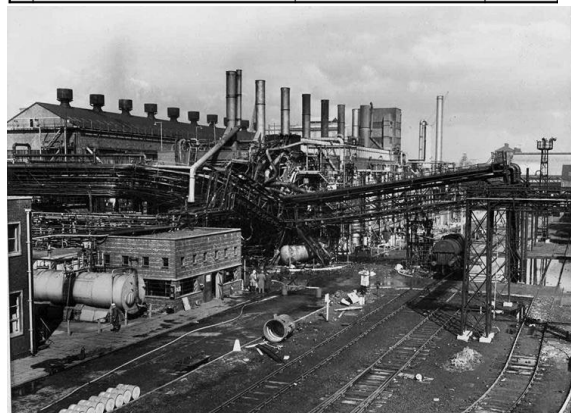
Fig 6. General View Looking North West
