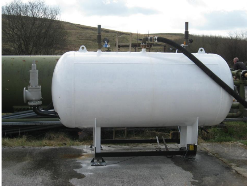
Figure 1. Reservoir used for valve testing under static conditions and showing M size valve in place.
