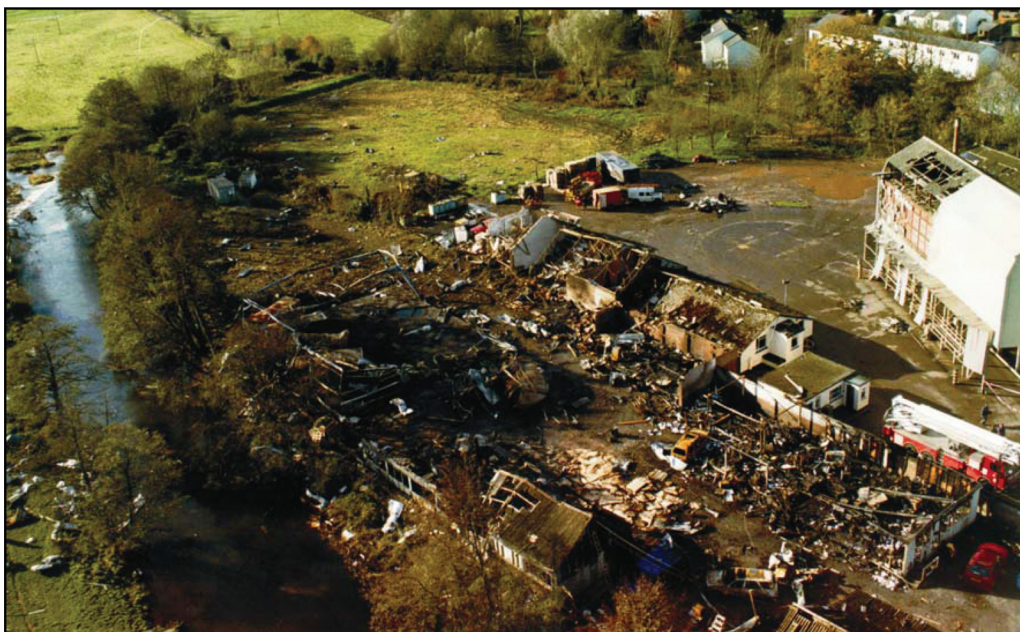
Figure 2. Uffculme fireworks complex after incident (Reproduced by permission of Aerial Photos)
