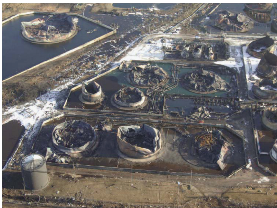
Figure 3. Aerial view to East of Bund A and its tanks. Tank T912 is in the centre foreground, T910, which was empty at the time of the incident, is to the right of T912 [ The Buncefield Incident, 11 December 2005; The final report of the Major Incident Investigation Board, Volume 1 (2008) p 1 ]
