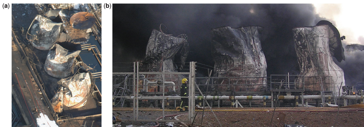
Figure 6. (a) Transfer tanks T601 to 603 as seen from the SW; (b) T601 to T603 as seen from the NE. These tanks are 6 m in diameter and 9.8 m tall. The tanks were obviously partially full at the time of crushing (Atkinson, 2010)
