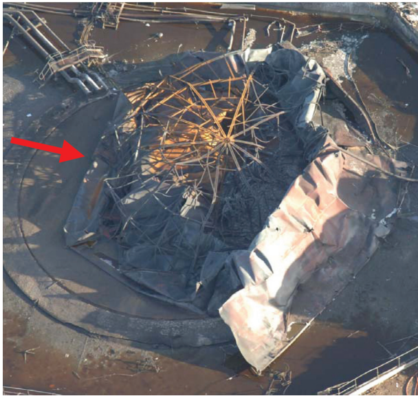
Figure 13. Tank 910 – the red arrow indicates the direction of explosion propagation
