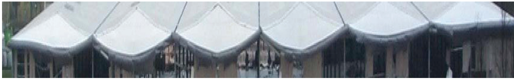
Figure 8. Variation in deformation of roof line on North face of WH1. Image digitally stretched (vertically)
