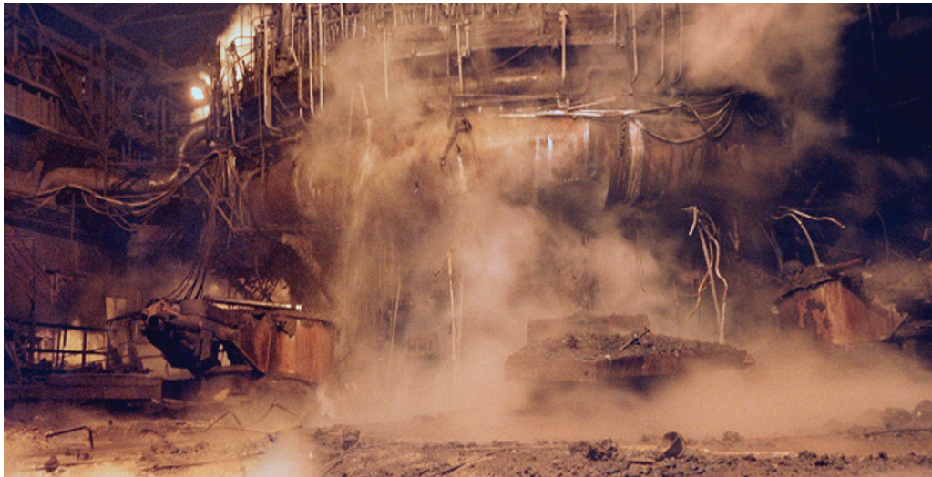
Figure 1. Blast furnace no. 5. picture taken from the cast house floor shortly after the incident
