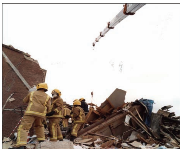
Figure 2. Elevated steel and concrete floor section
