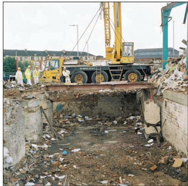
Figure 7. Showing floor section lifted back into place
