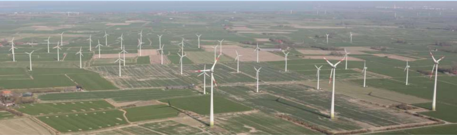
Lower Saxony generates a quarter of Germany's wind power and has an installed wind power capacity of 7,800 MW. It plans to increase this to 20,000 MW by 2050
