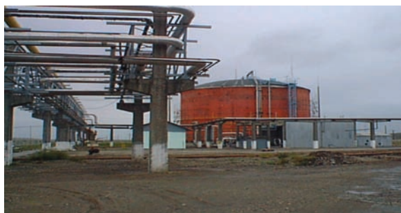
Figure 1. 13,000 t Ammonia storage tank at SOFERT SA
