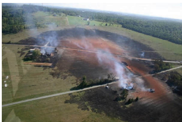
Figure 1. Gas pipeline incident in Virginia, USA in September 2008
