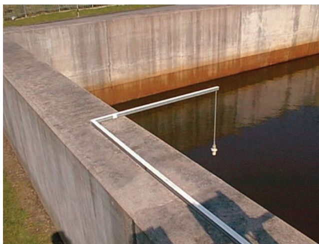
Picture 4. These ultrasonic sensors accumulate spiders and cobwebs and are difficult to clean and replace
