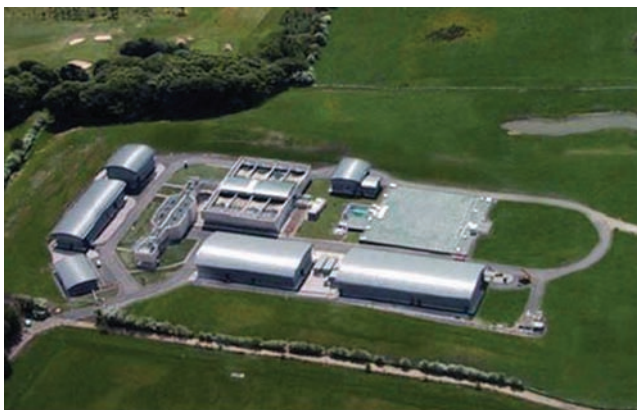
Picture 8. Lostock Water Treatment Works – our best water treatment works! Ultrasonic level sensor – how is it cleaned and replaced?
