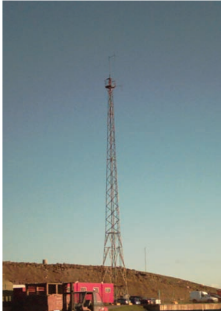
Figure 8. Transmitter mast at site E
