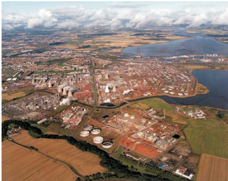
Figure 1. Photograph of BP Grangemouth complex
